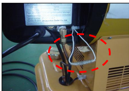
Picture 6 Inspection terminals for control device(PH5)
