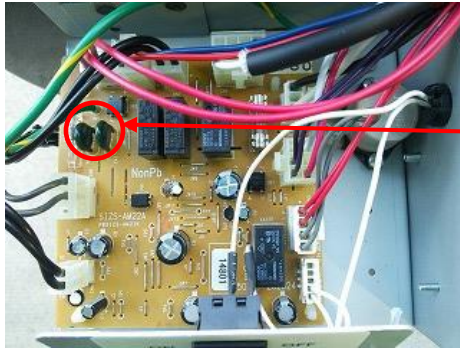
Picture 9 Inspection surge absorber (SA)
