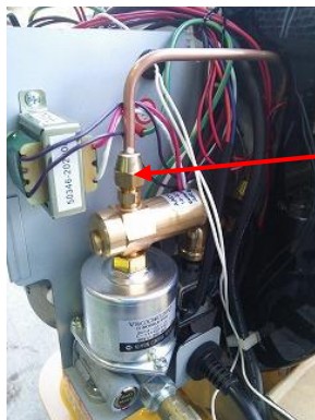
Picture 4 Inspection fuel pump
