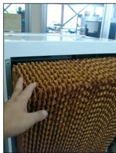
Pull out cooling element
